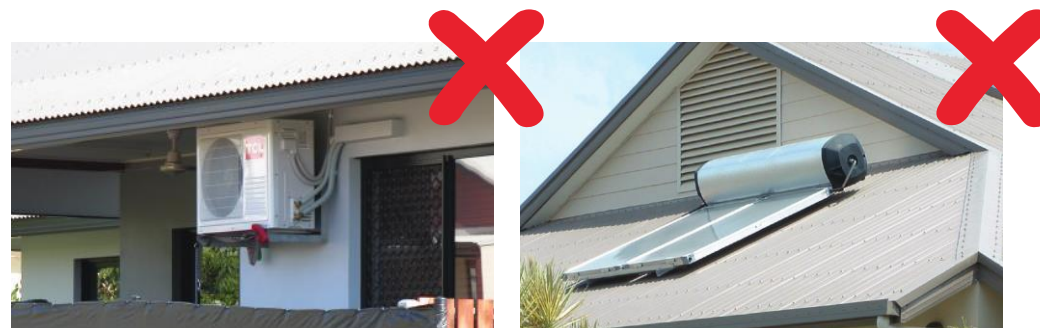
Minimise the visual impact on streets, parks and neighbouring houses when locating services such as air conditioning units, solar hot water systems and photovoltaic panels.
