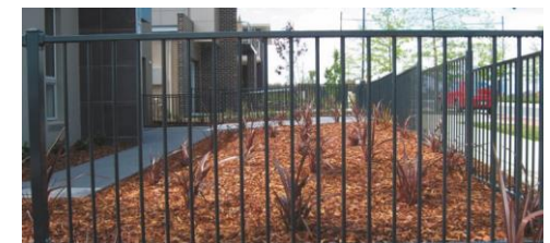
Square metal tubular dividing fence forward of the building line.
