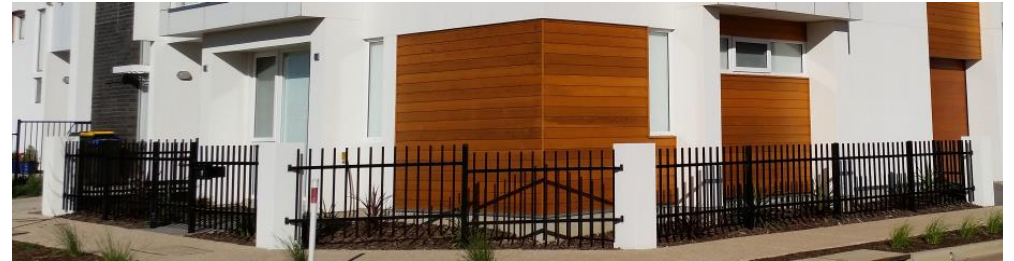
Example of fencing on corner allotments where the front fence continues along the secondary street frontage.
