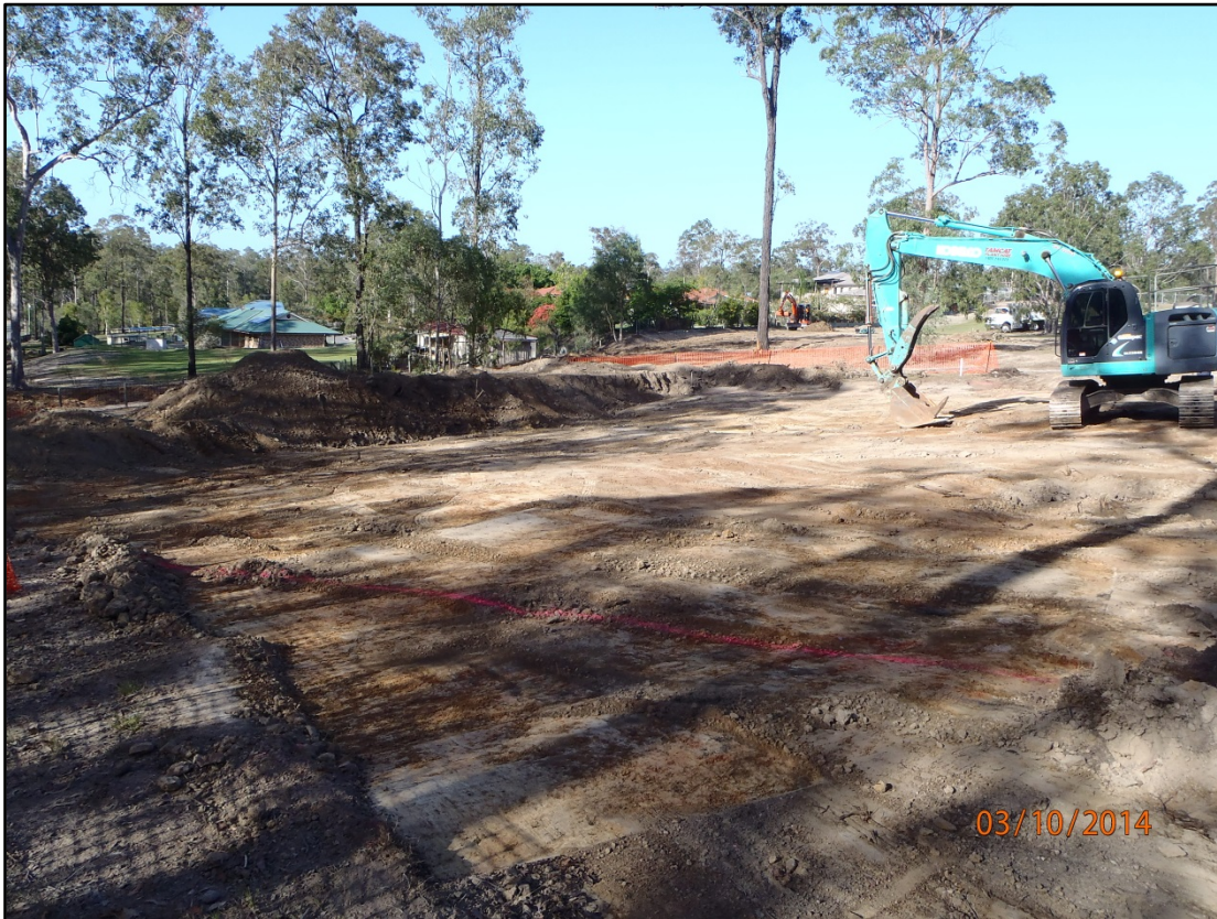
Figure 1: Subgrade preparation across building platform, facing south
