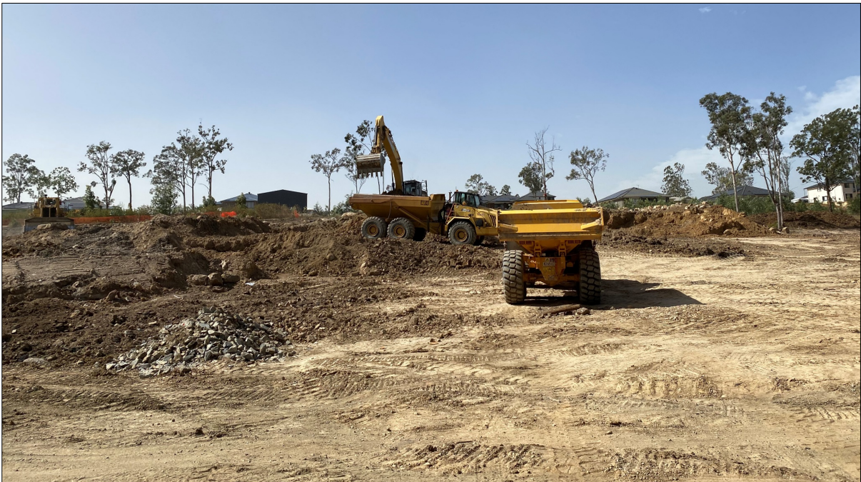
Figure 4 – Excavator and dump trucks, to move stockpiled fill material. (Taken 20/08/2020)
