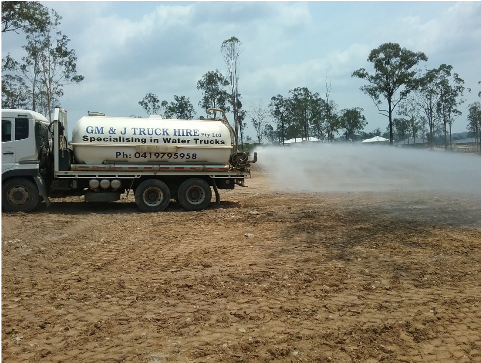
Figure 1 – Water truck moisture conditioning material prior to padfoot compaction. (Taken 10/12/2019)
