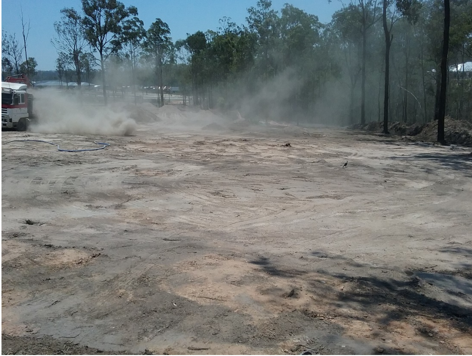
Figure 7 – Stripped area prior to compacted fill. (Taken 09/12/2019)
