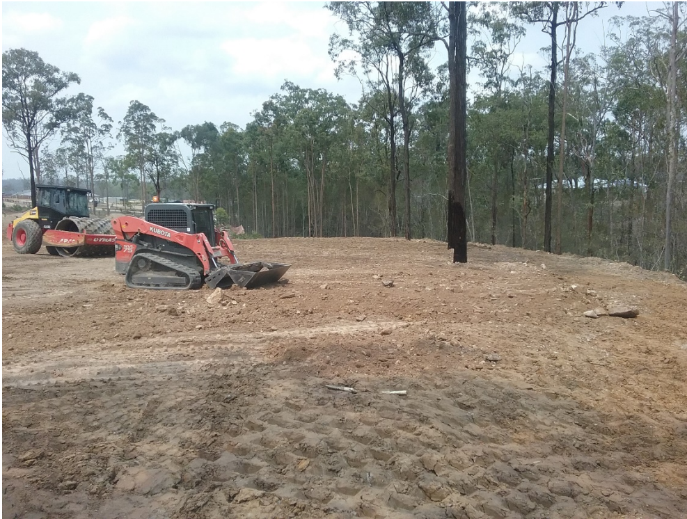
Figure 3 – Bobcat levelling placed fill. (Taken 09/12/2019)
