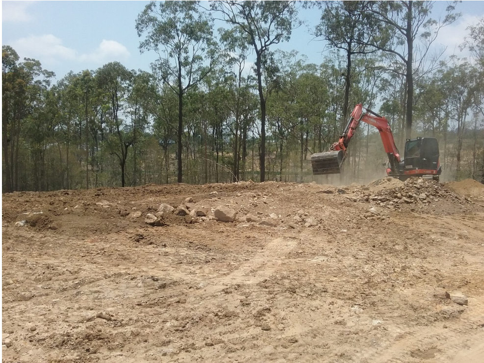
Figure 5 – Excavator placing and removing unsuitable rock (Taken 09/12/2019)
