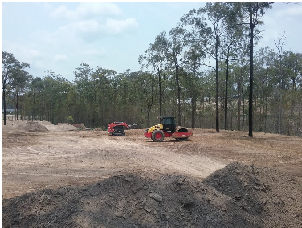
Figure 2 –Bobcat and padfoot roller placing and compacting fill. (Taken 09/12/2019)
