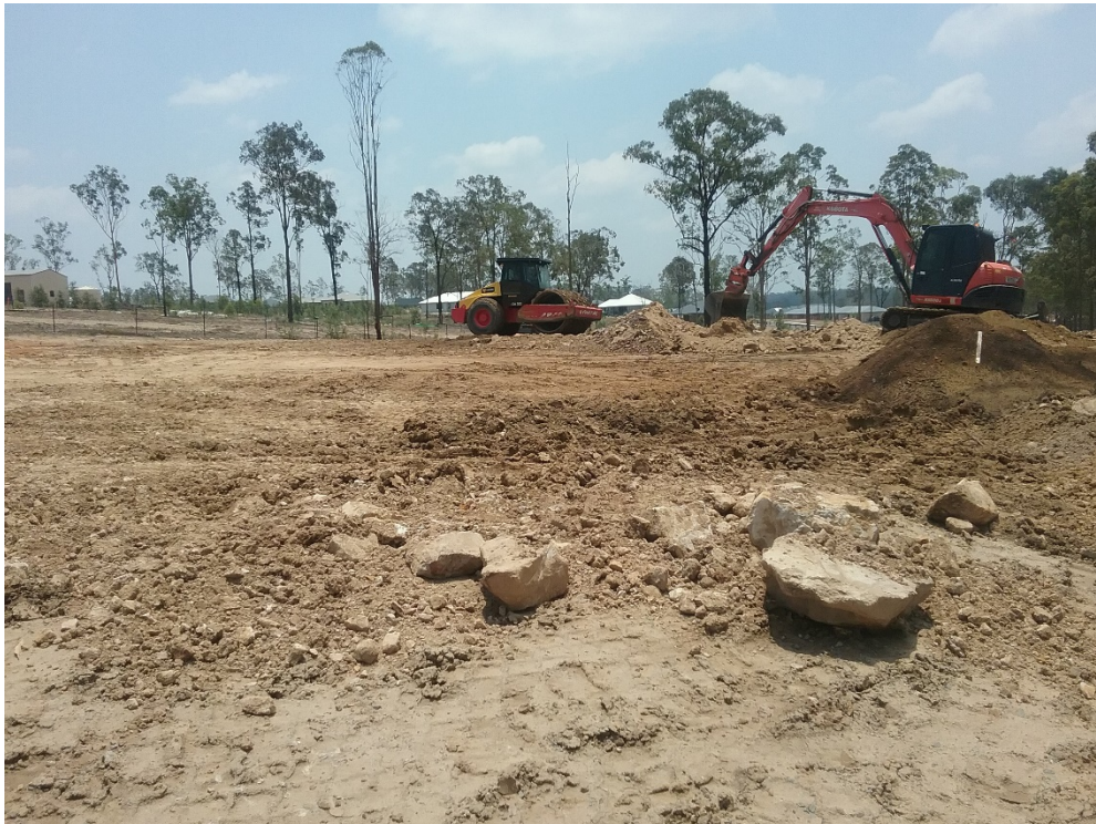
Figure 4 – Excavator placing fill and removing unsuitable size rock from fill. (Taken 10/12/2019)
