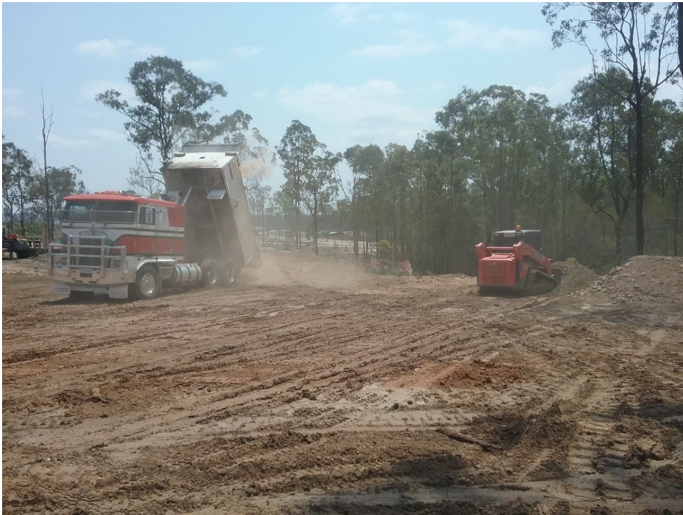
Figure 6 – Tip body truck and bobcat dumping and placing fill. (Taken 10/12/2019)
