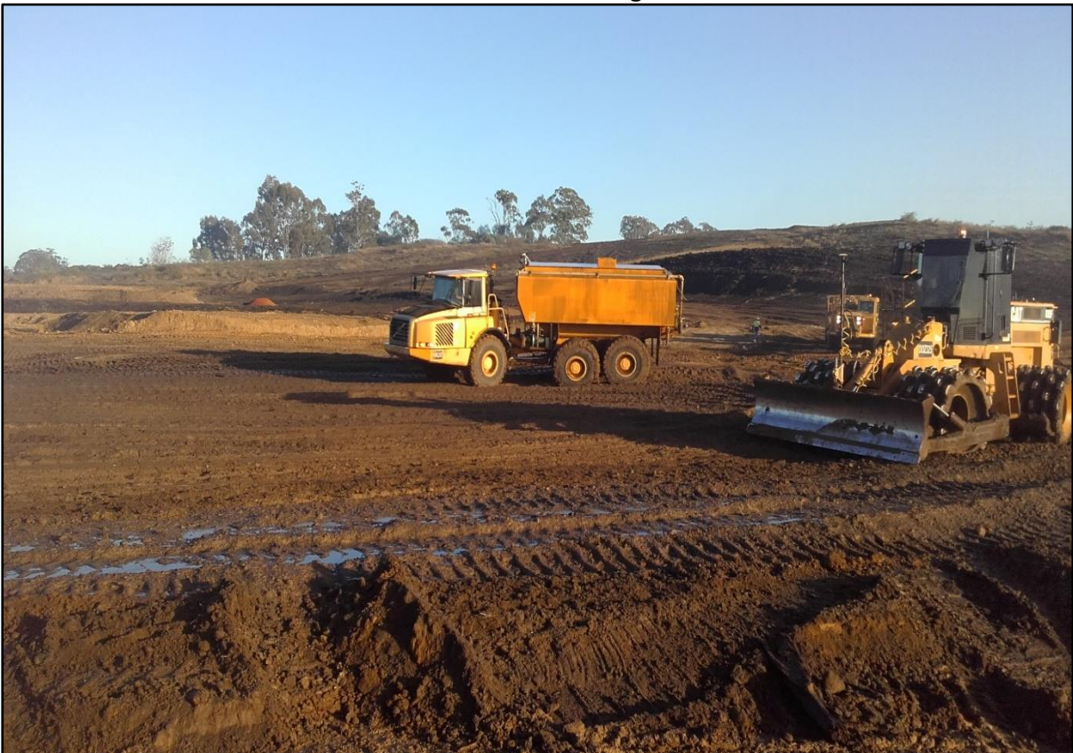
Picture 4: View of the Site During Construction
