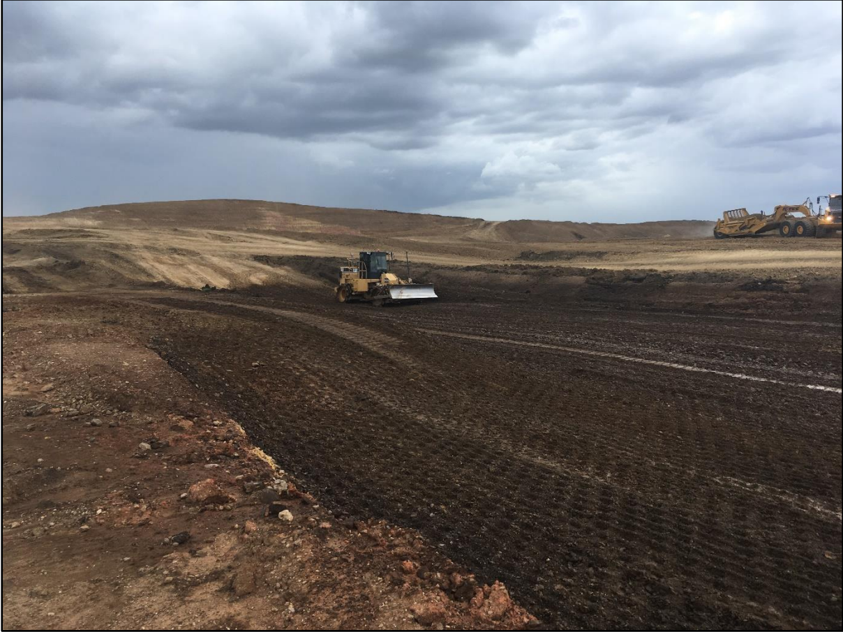
Picture 3: View of the Site During Construction
