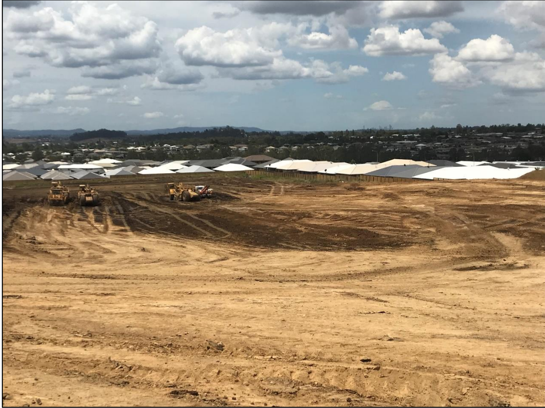
Picture 2: View of The Site During Stripping Operations
