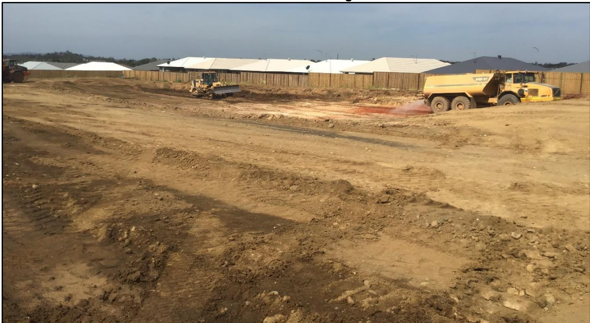
Picture 3: View of the Site During Construction
