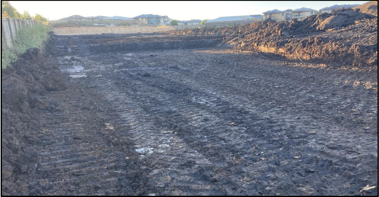
Picture 3: View of Pads at 1.2m Below FL
