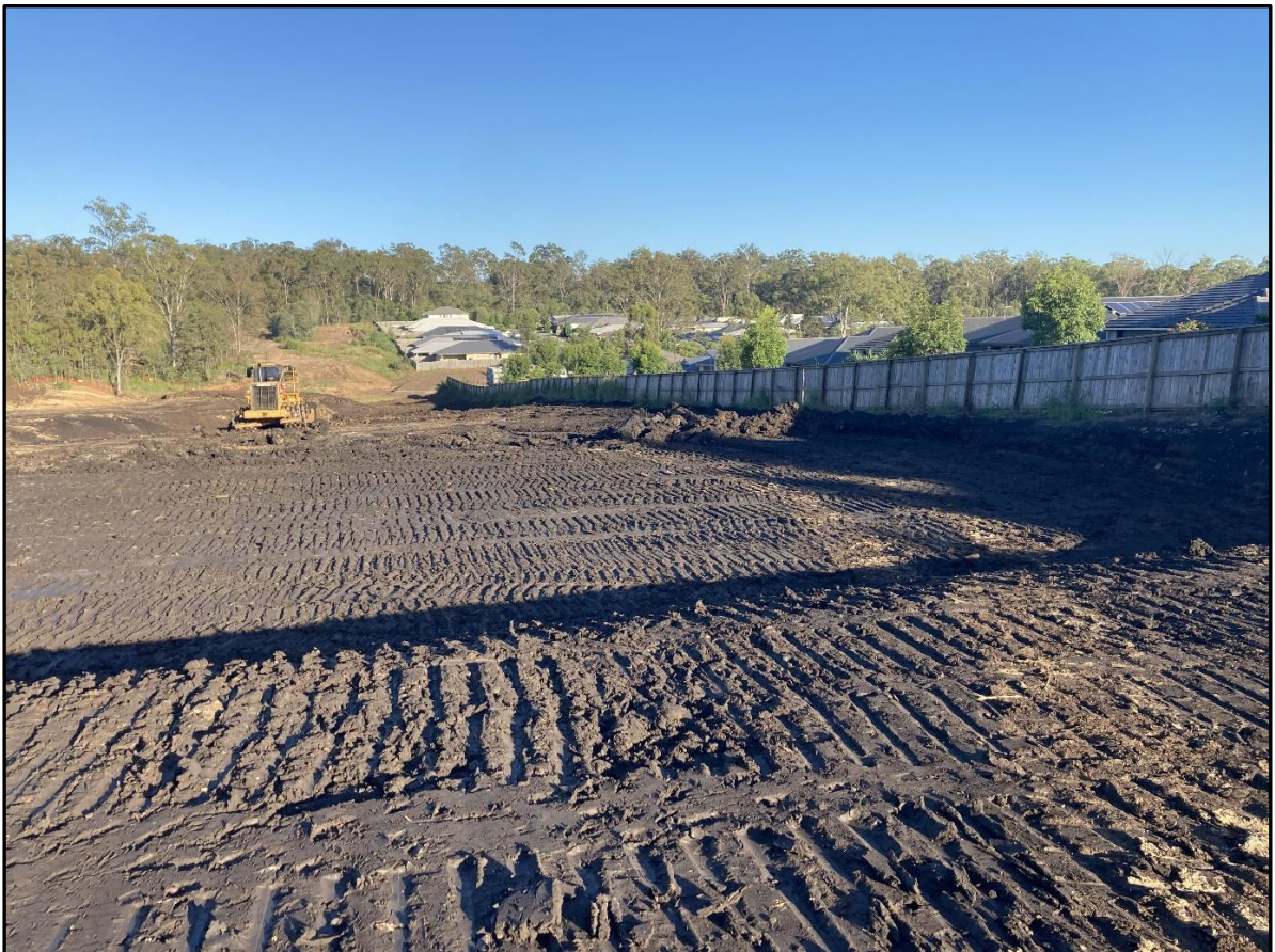
Picture 3: View of Pads at 1.2m Below FL
