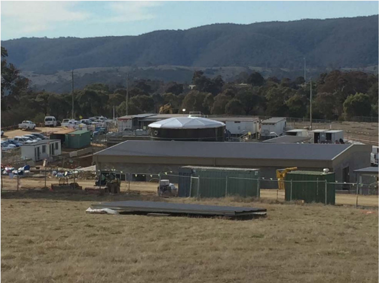
Figure 3-7 Existing recycled water tank at the WRP site (as viewed from the Googong sales viewing platform about 500 metres west of the WRP)
