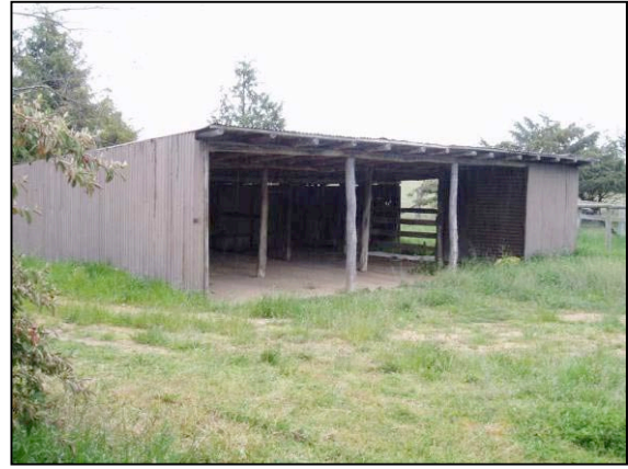
Figure 7.7 GH13 – Exterior view of shed
