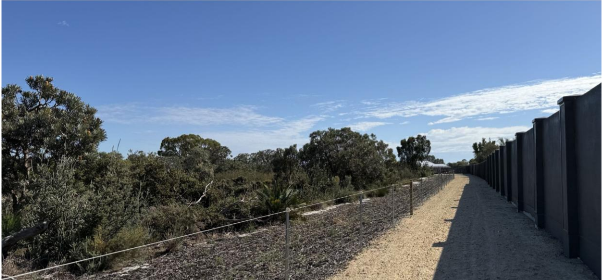
Plate 1: 16/04/2026 Constructed noise wall on the eastern boundary of Lot 102, permanent conservation fencing installed around conservation area and enviro-mulch installed along eastern boundary during this reporting period
