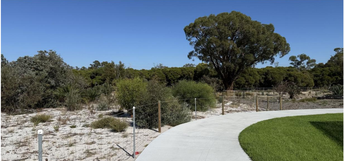
Plate 7: 16/04/2026 Designated paved walk path running along the conservation zone on the northeastern perimeter of the site, with conservation style fencing separating this zone from the park area
