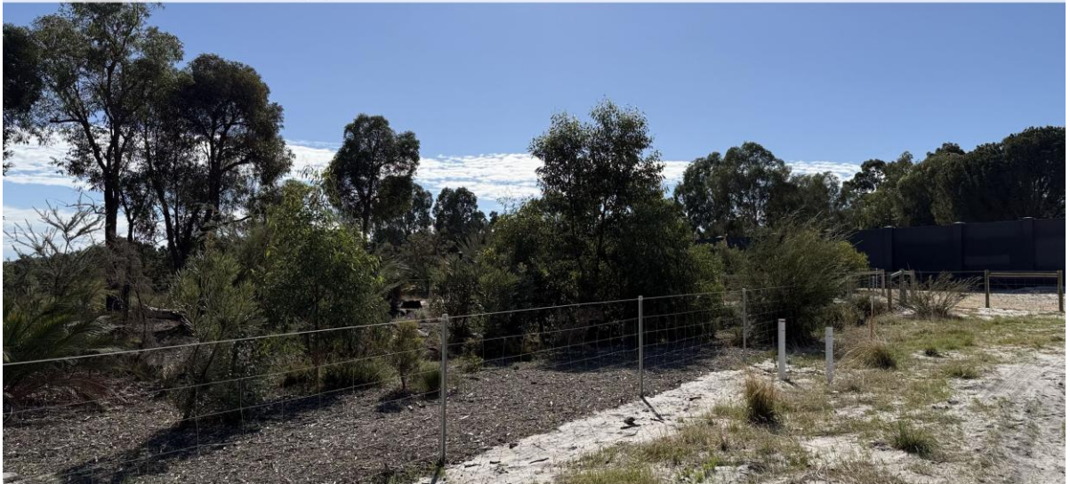
Plate 6: 16/04/2026 Permanent conservation fencing installed around conservation area and installation of enviro-mulch applied along the southwest boundary
