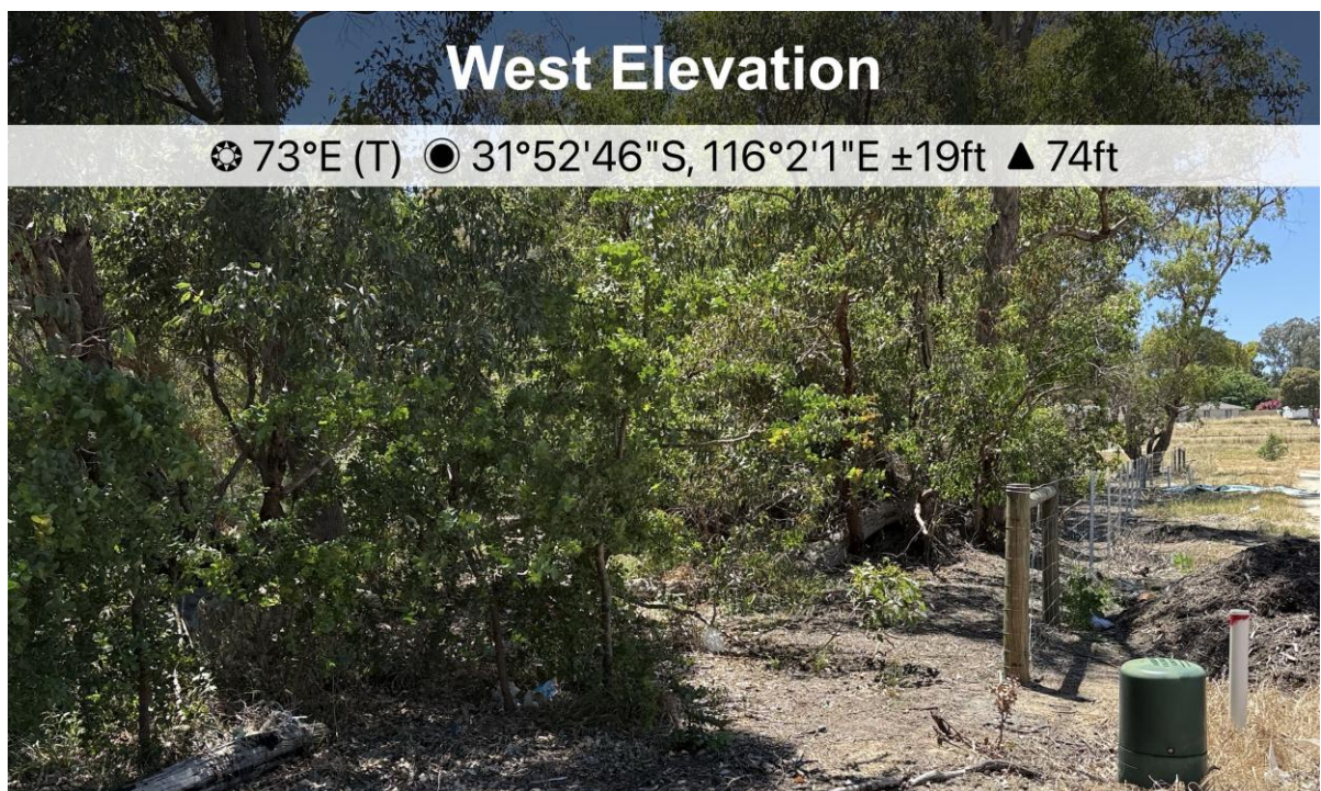
Plate 10: Photo of the fencing gaps identified in November 2025 that were subsequently fixed during this reporting period, as illustrated in Plate 11
