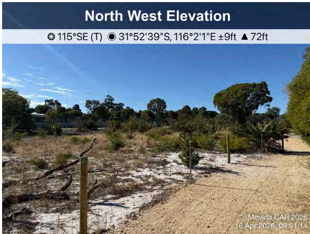
Photo 1: Conservation fencing installed (16/04/2026)
