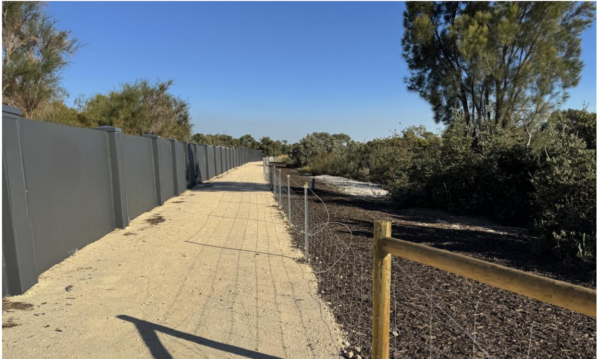
Plate 1: 28/04/2025 Constructed noise wall on the eastern boundary of Lot 102, permanent conservation fencing installed around conservation area and enviro-mulch installed along eastern boundary during this reporting period.
