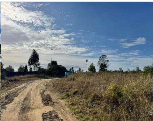
Figure 3. During Clearing Works:
