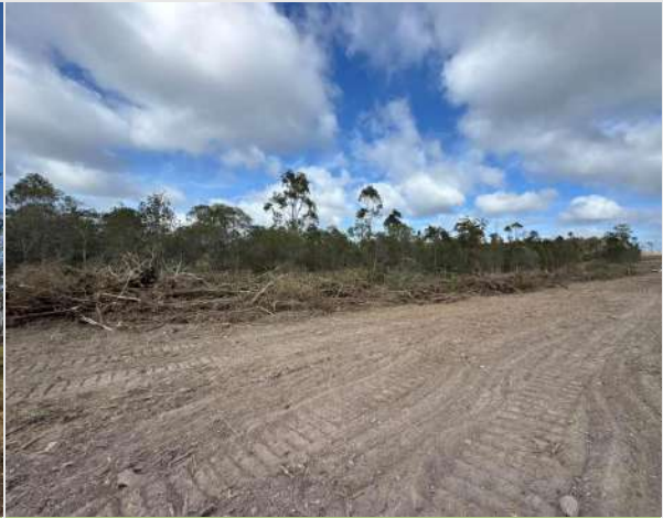
Figure 5. Post Clearing Works:
