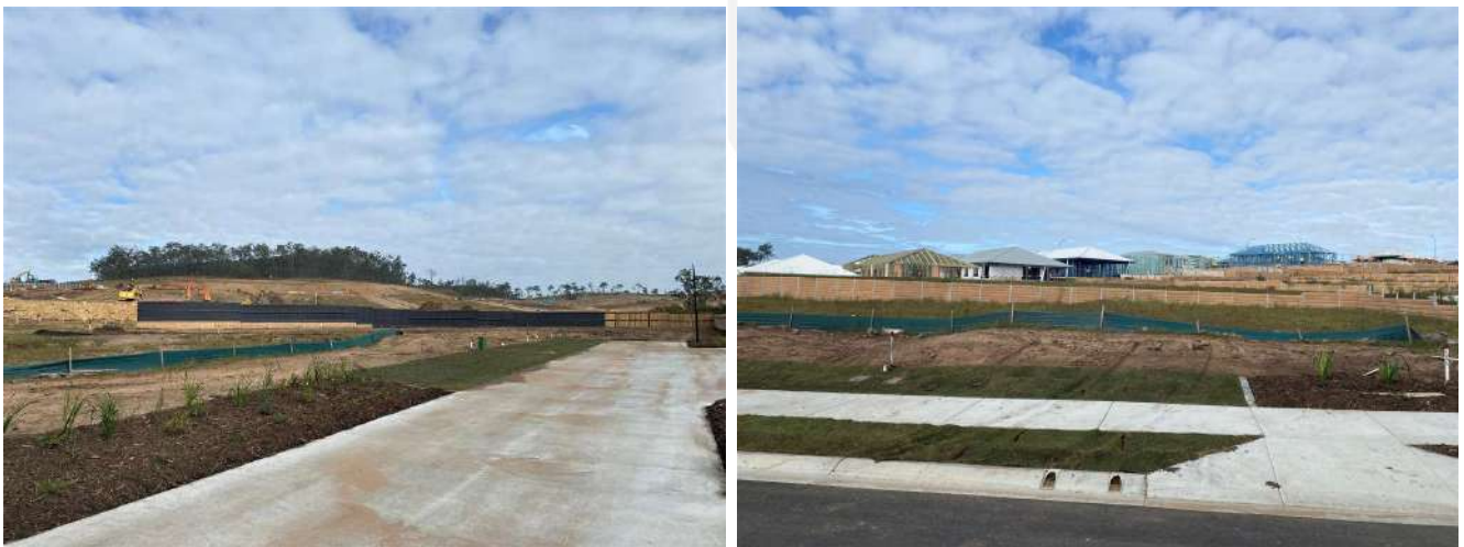
Photo set 1: Construction of residential land parcels and housing during the reporting period
