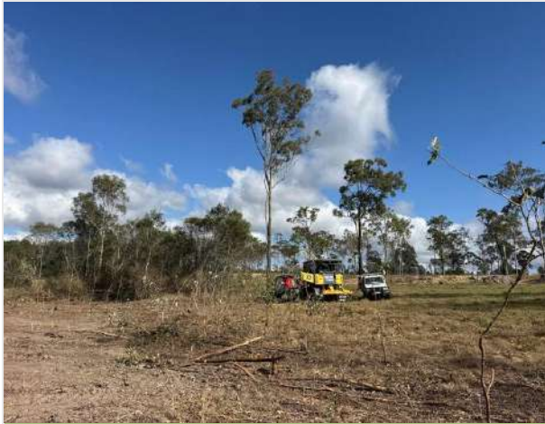
Figure 4. During Clearing Works:
