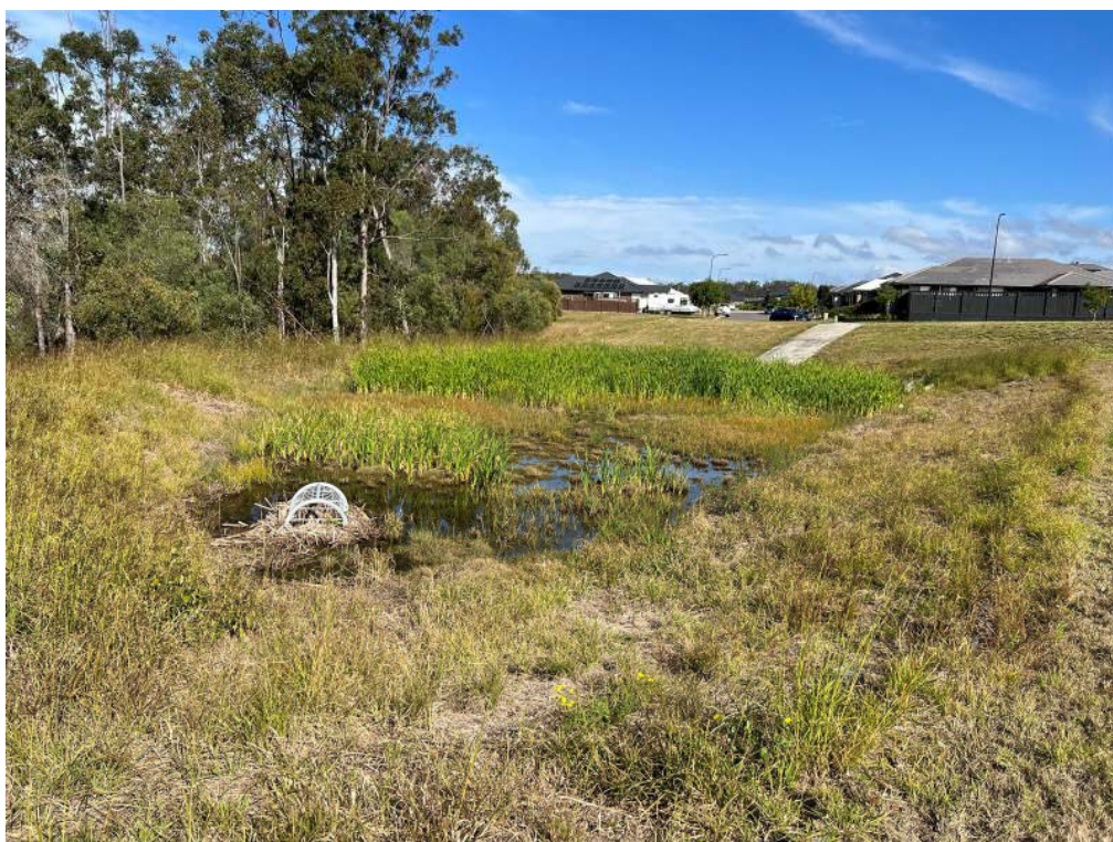
Photo 8: Established detention basin in south-west.
