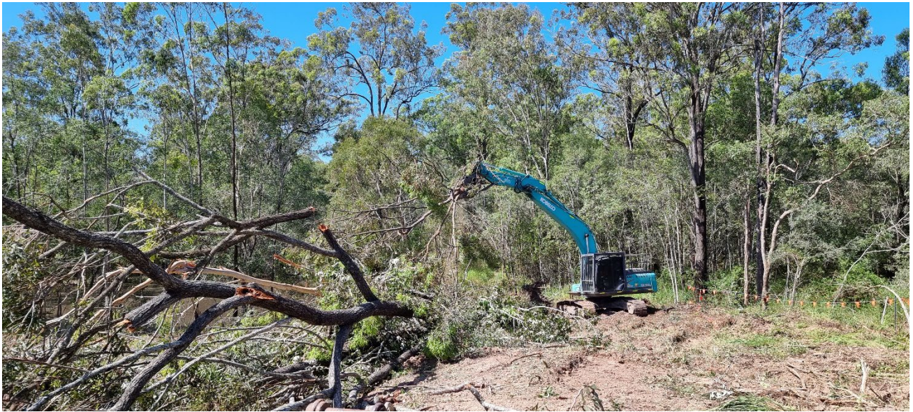
Photo 6 – Clearing with an excavator
