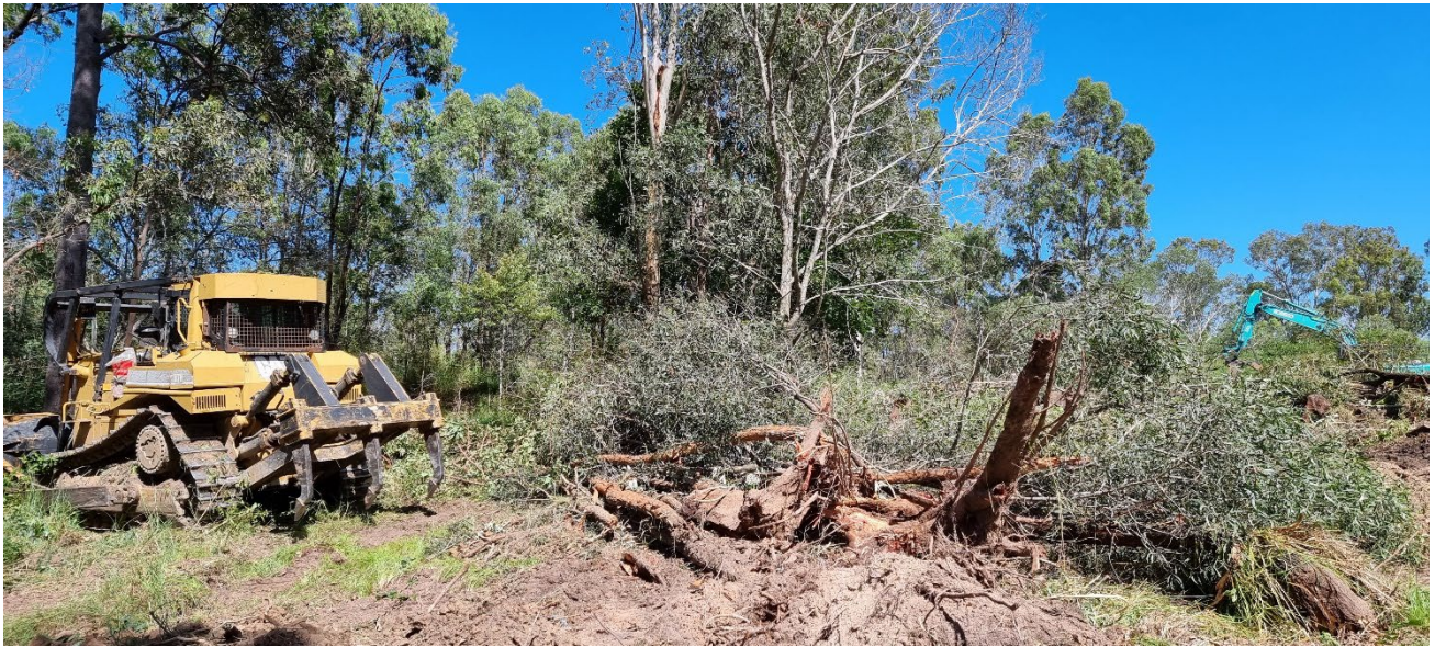
Photo 1 – Clearing with a bulldozer
