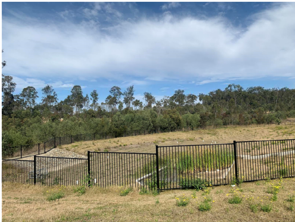
Photo 7: Detention basin in south-west created during the last reporting period.
