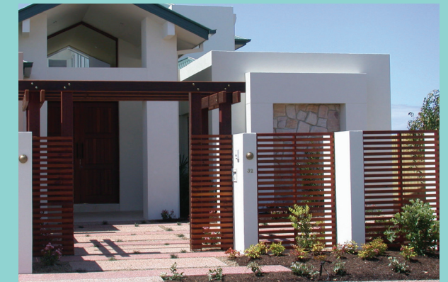
IMAGE 8 FRONT FENCING – EXAMPLE 2 Maximum height is 1200mm measured from ground level. Alternative dressed timber fence that reflects the dwelling design.
