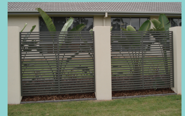
IMAGE 9 FRONT FENCING – EXAMPLE 3 Maximum height is 1200mm measured from ground level. Appropriately detailed glass and/or glass infill or powder coated aluminum.
