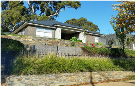
Complying example of retaining walls with approved materials
