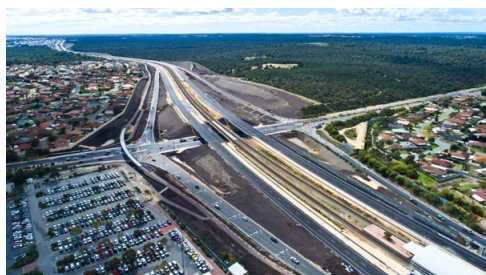
Mitchell Freeway extension Courtesy of Main Roads Western Australia
