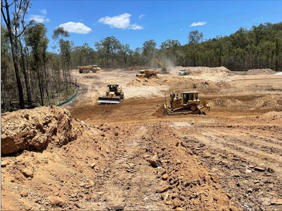
*Figure 1 – Heavy machinery placing and spreading out fill. (Taken 05.11.2020)*
