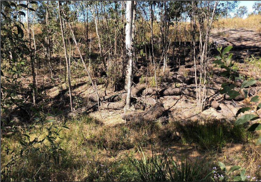
Photo 3: Bank stabilisation requiring minor maintenance.
