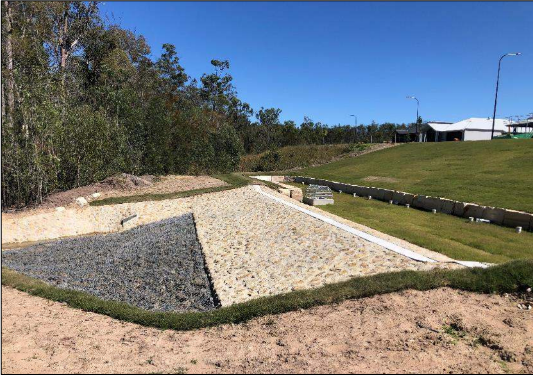
Photo 2: Detention basin in south-west.
