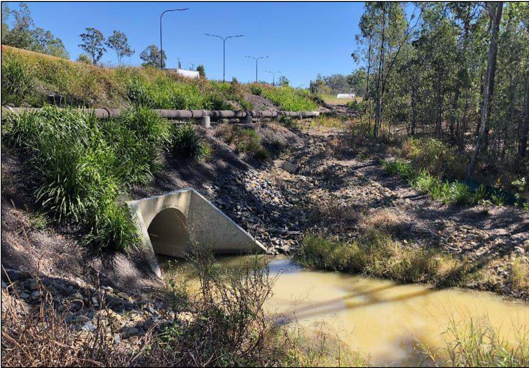
Photo 5: Rehabilitated area on the eastern side of Flagstonian Drive bridge crossing.
