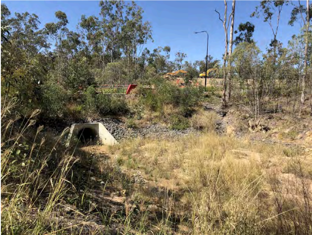
Flagstone Bridge culvert
