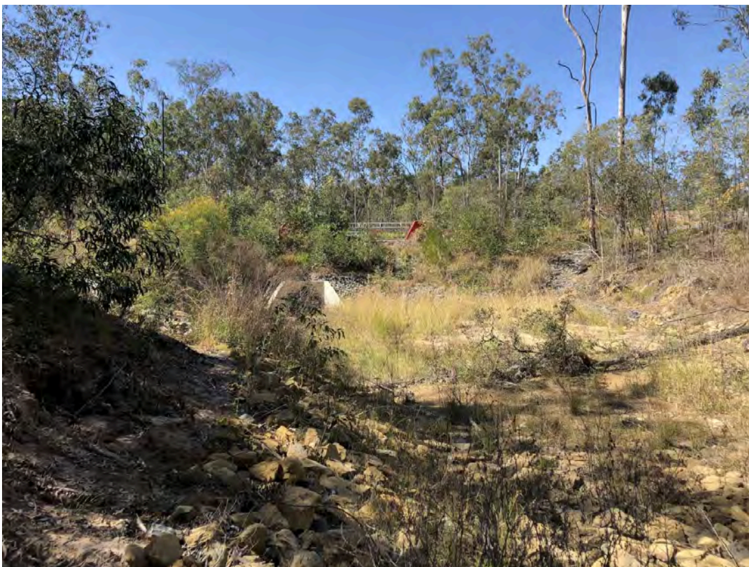
Flagstone Bridge (view from creek bed)
