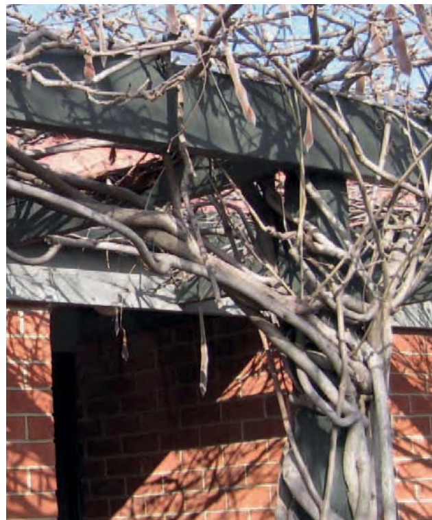
Vines and creepers act as ladder fuels.
