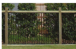
Timber & infill 'pool fencing'
