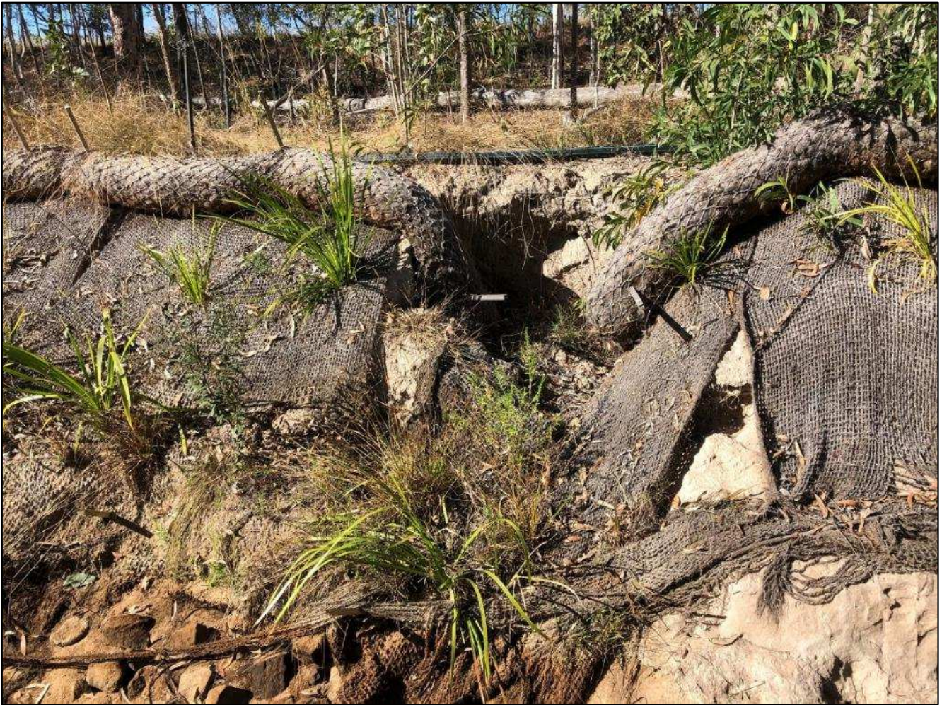
Photo 12: Matting requires attention in sections along Sandy Creek tributary.
