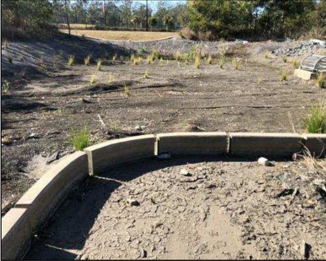
Photo 6: Existing condition of detention basin.
