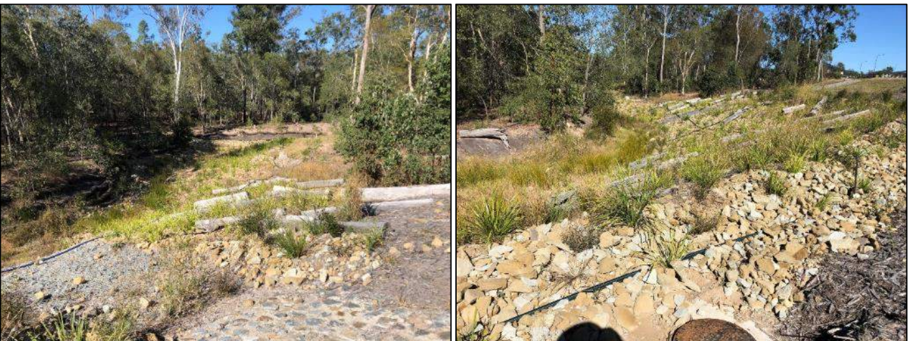
Photo set 19: Rehabilitation works along creek.
