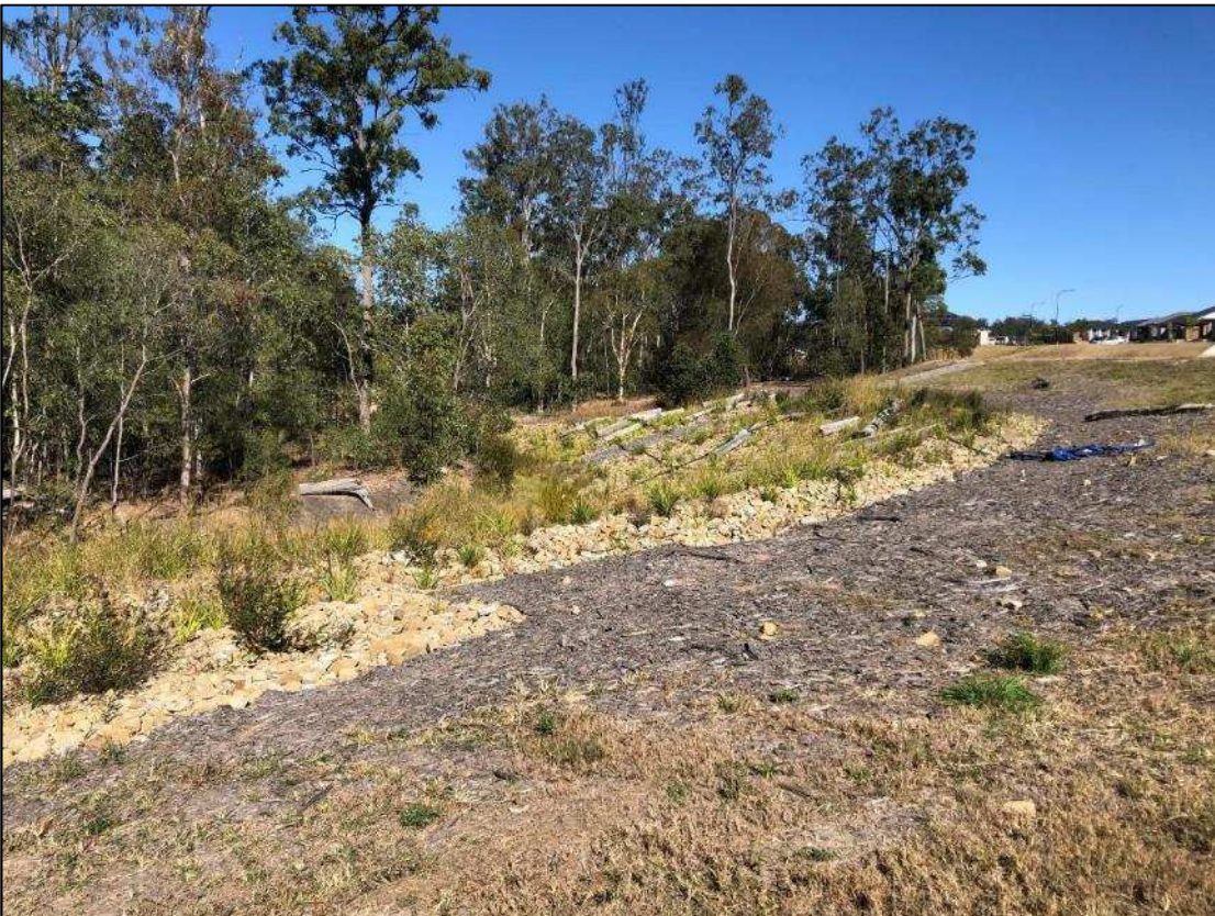
Photo 21: Bank rehabilitation and stabilisation works.
