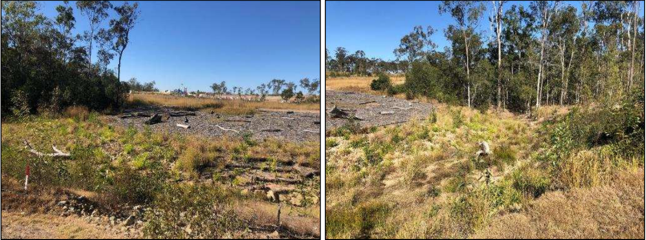
Photo set 17: Bank stabilisation works and in-stream rehabilitation and stabilisation works.
