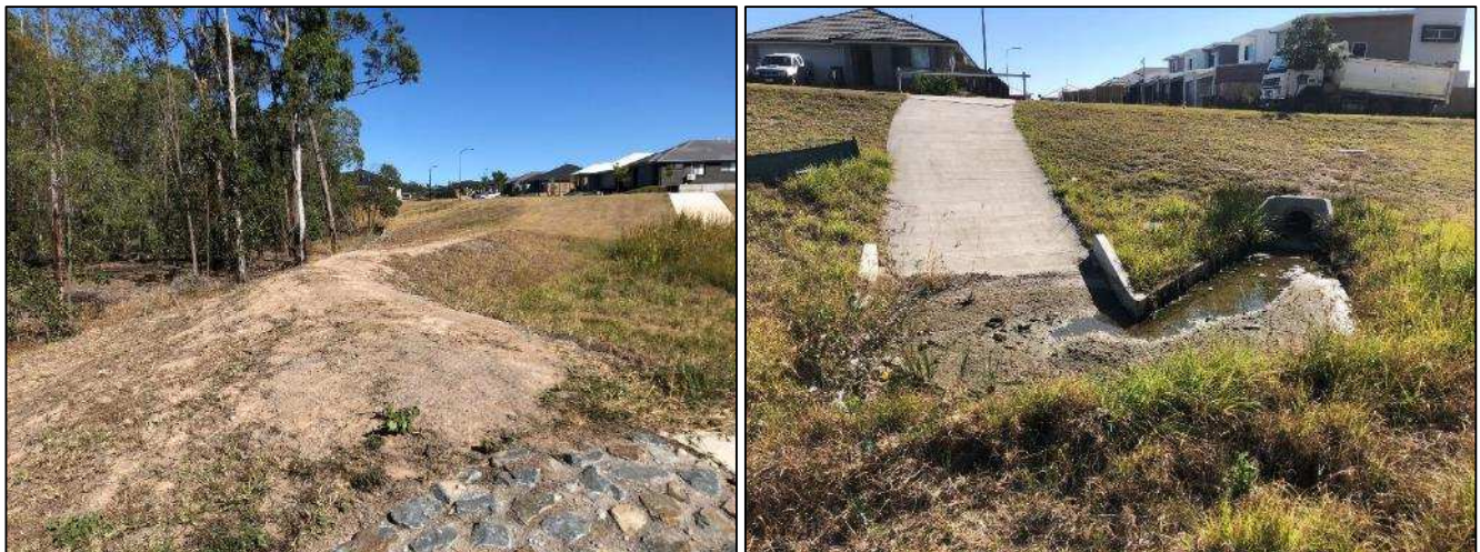
Photo set 13: Bund (left) and sediment build-up within drainage area north of Sandy Creek tributary (right).
