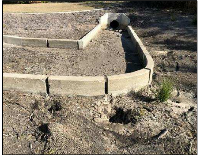
Photo set 7: Erosion damage to rehabilitation matting within detention basin.
