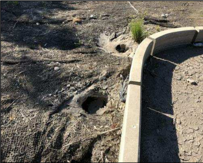
Photo set 7: Erosion damage to rehabilitation matting within detention basin.
