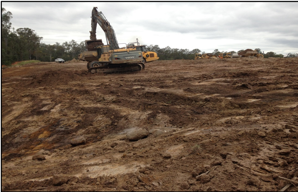
Picture 2: View of the Stripped Surface Prior to Filling Operations
