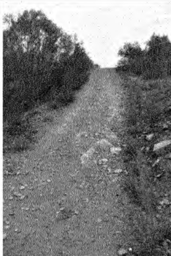
DSC 3768: Minor wheel rut erosion
