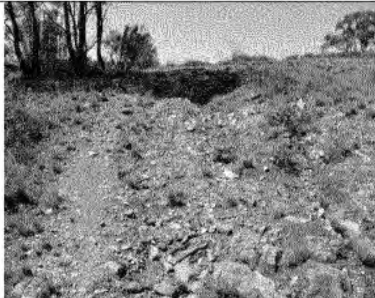
DSC 3823: Moderate-sloping sections upslope of the river flats require permanent drainage structures
