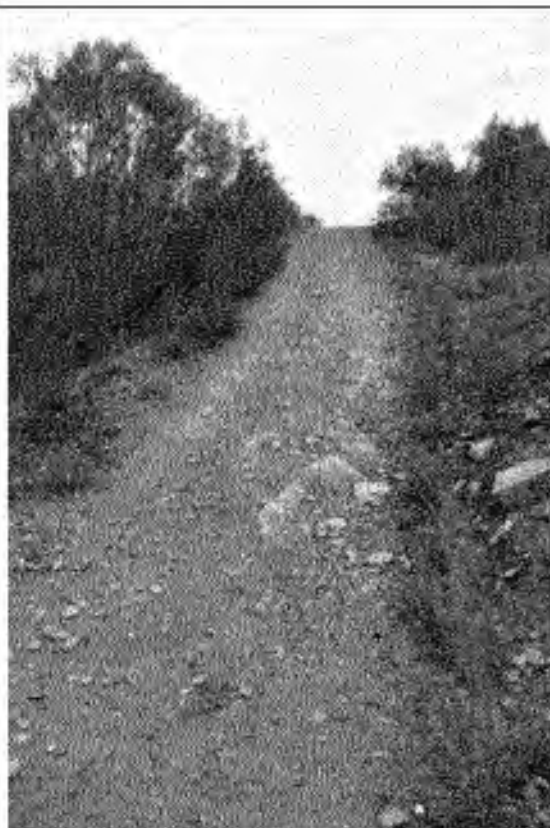
DSC 3768: Minor wheel rut erosion
