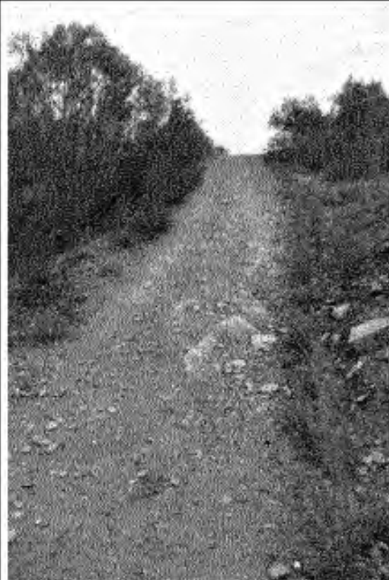
DSC 3768: Minor wheel rut erosion
