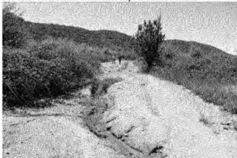
DSC 3837: Minor erosion on sloping sections of trail
