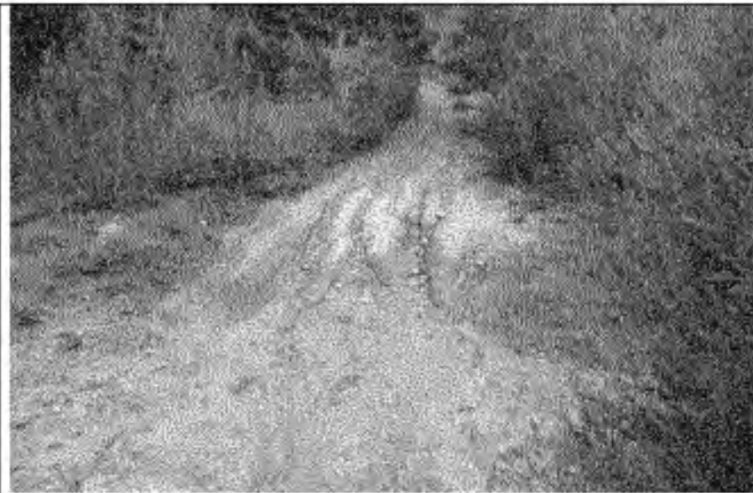
DSC 3770: Wheel rut erosion and deposition in channel of crossover
