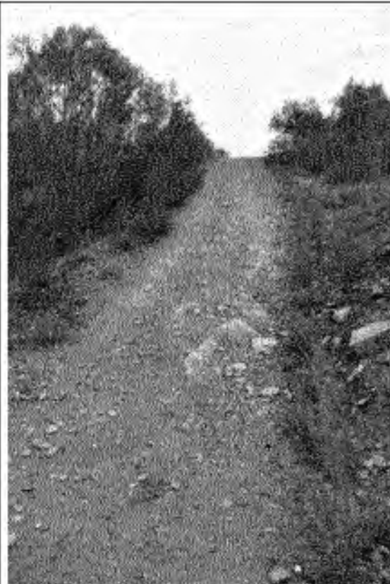
DSC 3768: Minor wheel rut erosion
