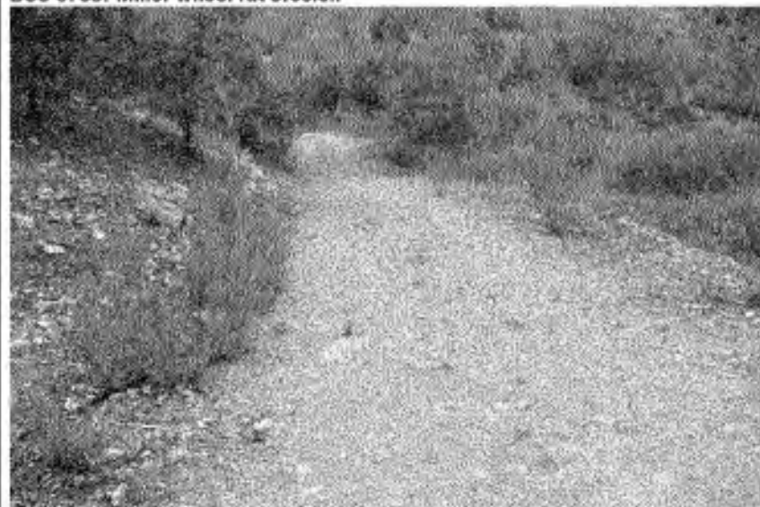
DSC 3769: Trail in general good condition with all-weather surface
