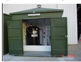
A typical contained chemical dosing unit is shown in Figure 3-2.
