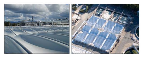
Figure D-8 FRP Arc Span Anaerobic and Anoxic Zone Covers
