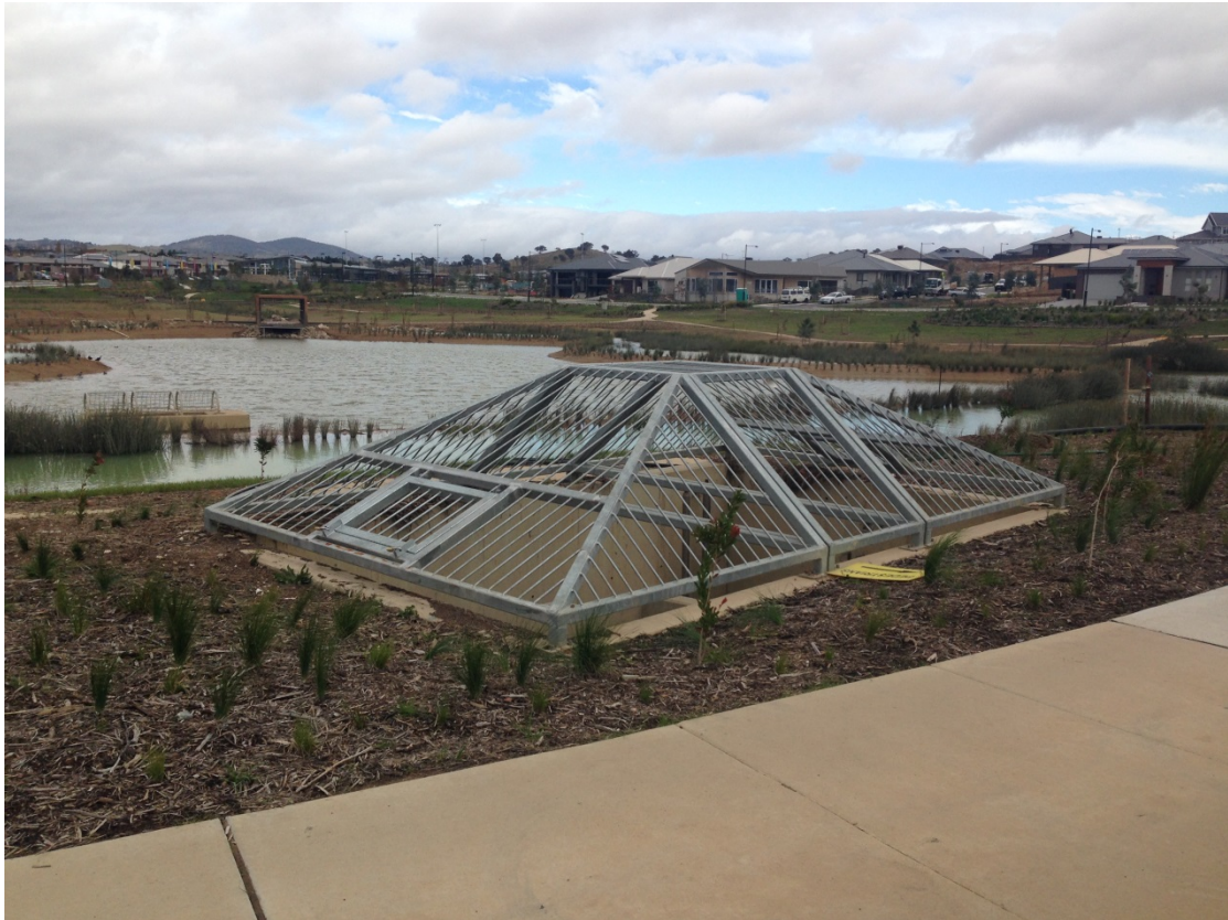
Plate 3 Outlet structure at Beltana Park
