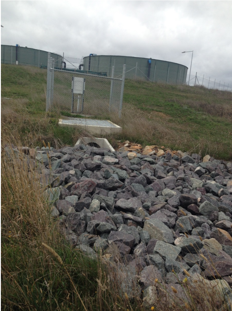
Plate 2 Energy dissipater/scour protection at interim reservoir discharge point
