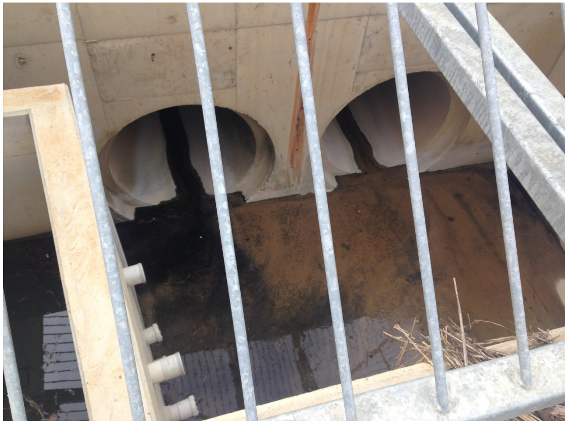
Plate 4 Inside of outlet structure, showing 1650 mm diameter reinforced concrete pipes that transfer recycled water to Googong Creek
