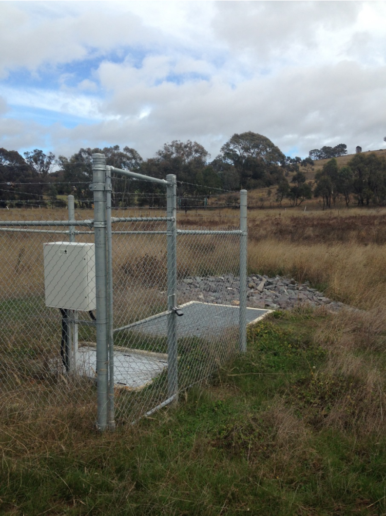
Plate 1 Flow meter and ORP analyser, housed inside pit (foreground) with weir pit to full pipe in mid-ground
