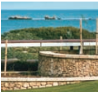
New boardwalk, Burns Beach Estate.
